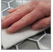
Allow grout to harden for about 20 to 30 minutes. Using a slightly damped white scrubbing pad, loosen up all excess grout over the tile with a circular motion. Do not add water before everything is well loosened up.
