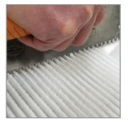
Apply an adhesive layer using the notched side of the trowel ridge in a straight-line directional pattern to achieve an even spread. For walls, maintain ridges running in a horizontal directional pattern.
