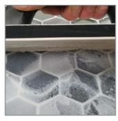
With a firm to medium sharp-edged rubber float, force grout diagonally into the joint at a 45° angle, ensuring that the grout is wellcompacted, free of voids and pin holes, and filled flush with the tile or stone edge.
