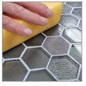
Then, using a slightly damped sponge (not wet), gently wipe excess material from the surface using light and delicate diagonal passes. Change water and rinse the sponge frequently. Keeping the water and sponge clean will achieve better joint color uniformity.
